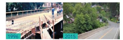
In US FRP was first manufactured in 1984 by the Kodiak Company. It was designed for applications where concrete is exposed to water, salts and other chemicals. The first vehicular structure built using FRP was Mckinley Ville bridge in 1996.
